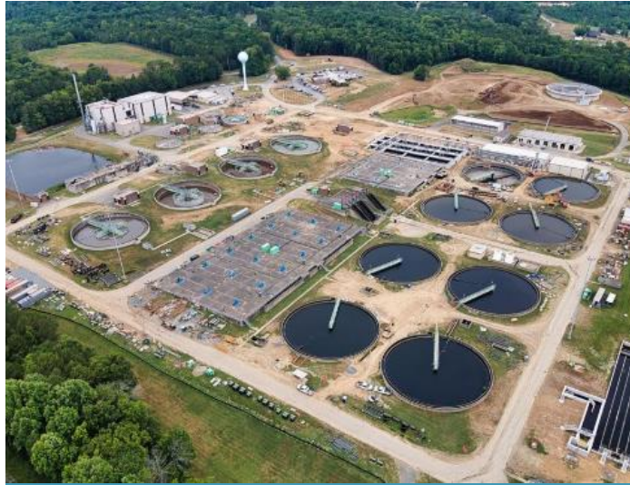
Rocky River Regional WTP
